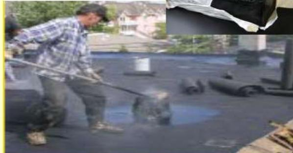
**VECCHIO SISTEMA DI POSA CON SPALMATURE DI BITUME (2006, tetto USA)**
